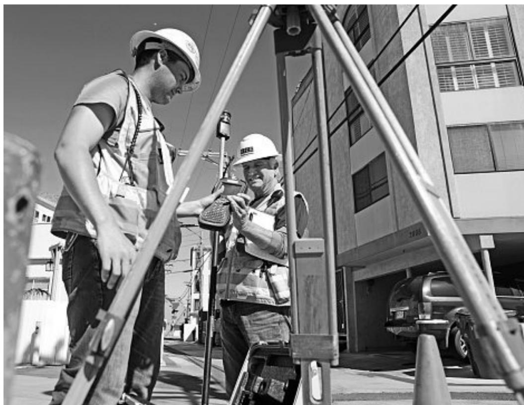
Dustin Gardner (left) and Paul Knox of Rick Engineering use a data collector to compile the measurements they collected using laser technology to create a topographic map.
